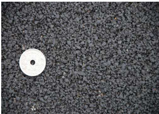
Rys. 10.13. Nawierzchnia jednowarstwowa (DVS-DRI Super Quiet Traffic International search for pavement providing 10 dB noise reduction, Danish Road Institute Report nr 178, 2009)
